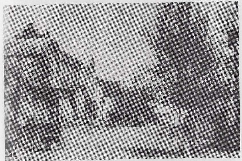
High Street in Millhousesen (now "The Main Street"). Buildings before fire in 1908.
